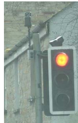
Plate 4. Close up of MOVA mounted on the pedestrian crossing
